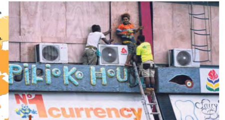
Locals in Vanuatu boarding up their shops in preparation for Cyclone Harold on April 6. This is to prevent their windows from breaking and water flooding the building.
